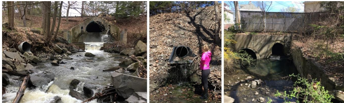
Figure 2: Examples of pipes that empty into the channel of the Hans Groot Kill. Left: Site HGK-2, with a tunnel and pipe outfalls at center and a pipe outfall at left. Center: Site HGK-5 Pipe, which commonly has the highest Enterococci levels. Right: Site HGK-7, the upstream end of the exposed HGK, where the Sheridan Avenue (left), The Plaza (center), and Rugby Avenue (lower right) storm sewer outfalls provide source water for the stream.
