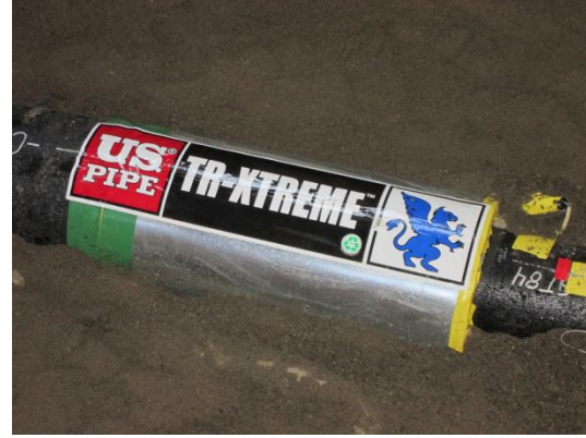
Figure 7.3. Pipe Joint with the Protective Shielding
