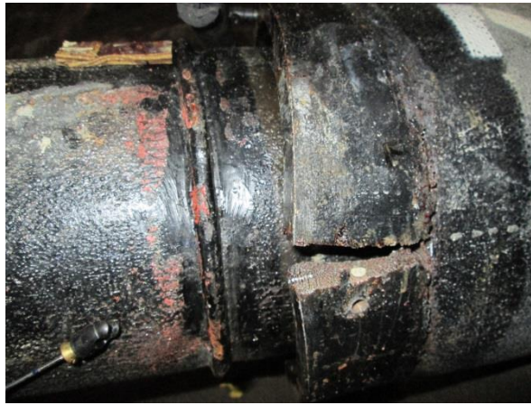
b) Elevation View of the South Joint from the West Springline
