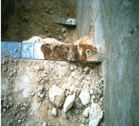
Figure 29. Corroded reinforcement
