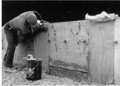
Figure 18. Geotextile joint cover
