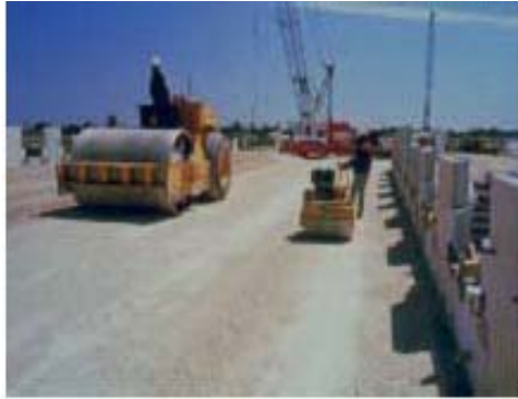
Figure 14. Compaction equipment roller
