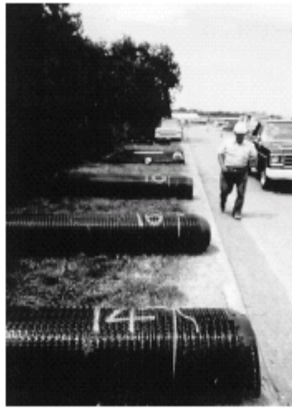
Figure 5. Inspect reinforcing elements
