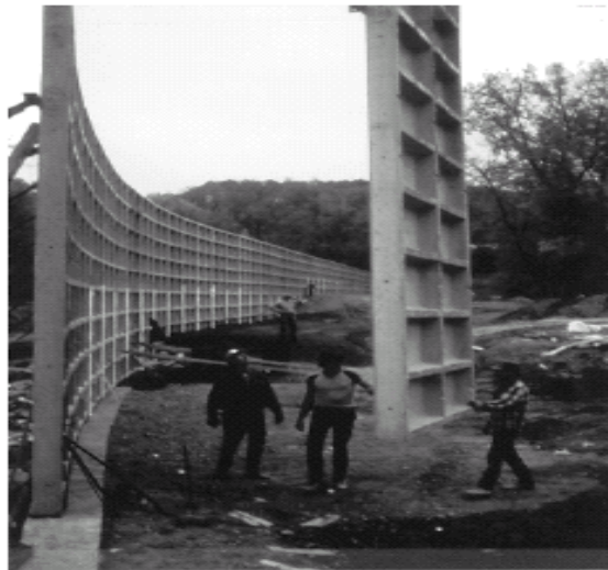
Figure 11. Setting first row of precast facing elements
