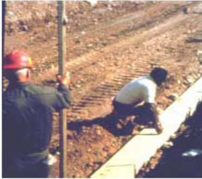
Figure 6. Leveling pad leveling pad
