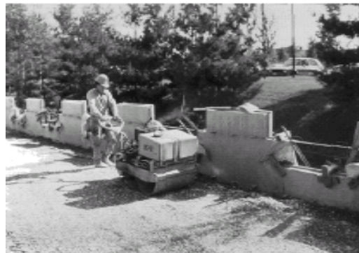
Figure 16. Lightweight equipment @ 1 m from face
