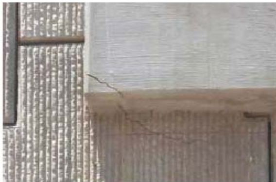
Figure 21. Cracked panel and cheek wall Figure 22. Tension break in cheek wall
