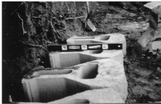
Figure 10. Checking facing element batter and alignment
