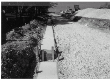
Figure 8. Concrete leveling pad leveling pad
