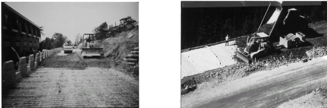
Figure 13. Placement of reinforced backfill
