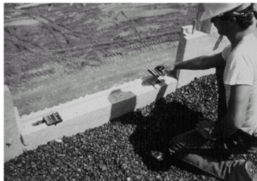
Figure 19. Neoprene bearing pad
