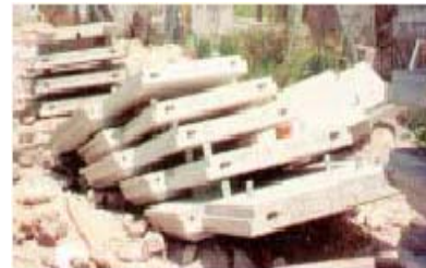
Figure 4. Improper panel storage
