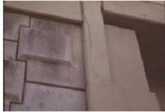
Figure 21. Cracked panel and cheek wall Figure 22. Tension break in cheek wall
