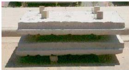
Figure 3. Proper panel storage
