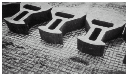
Figure 9. Compacted gravel leveling pad
