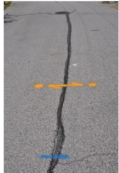
Figure 1 Crack sealing after several years
