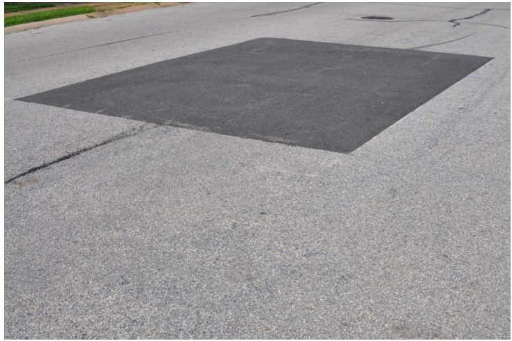
Figure 2 Pothole or distress patching
