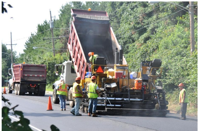
Figure 5 Pavement overlay of a milled surface
