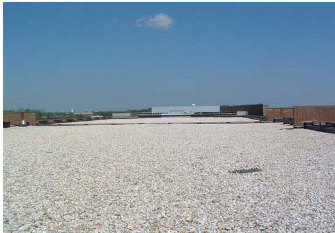
Figure 3. Highway Administration Building Roof
