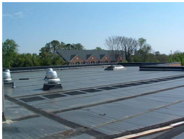
Figure 2. Richards and Robbins Building Roof
