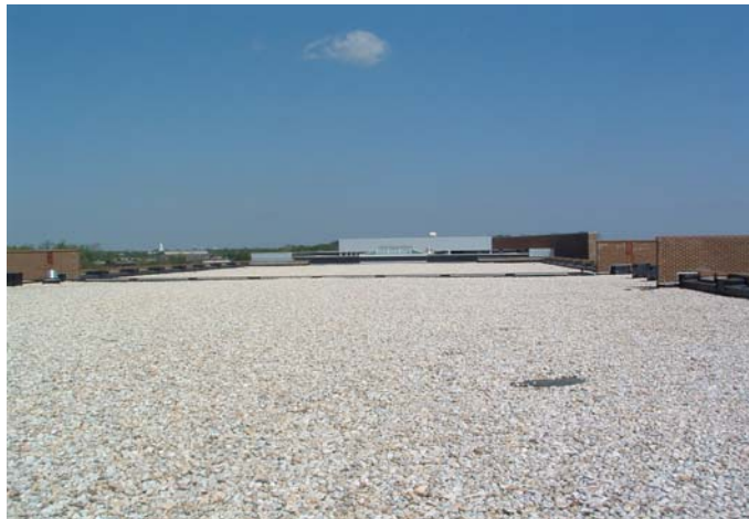
Figure 3. Highway Administration Building Roof
