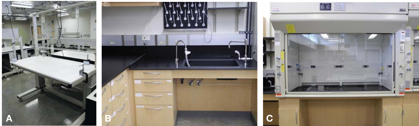
Figure 1. Wet Laboratory Work Triangle in ABIL with Automatic Adjustable-Height Lab Bench (A), Wheelchair-Accessible Lab Sink (B), and Wheelchair-Accessible Fume Hood (C).
