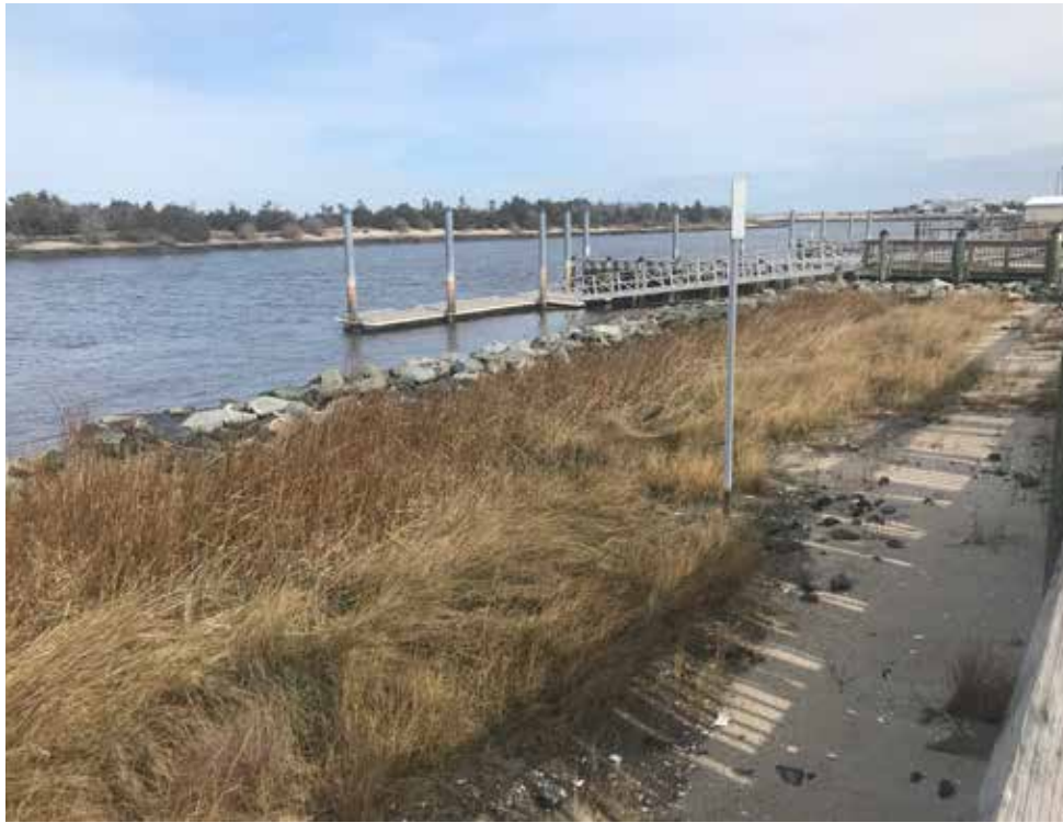
Figure 6: Marsh planting behind rock toe sill at DNREC field office; see Roosevelt inlet in the background.
