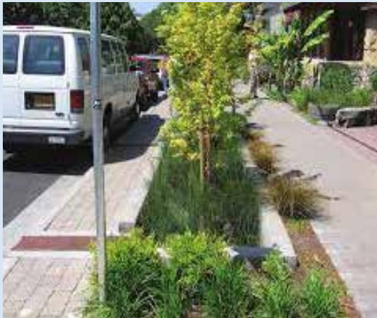
Image: Sidewalk constructed with permeable pavement via DNREC.
