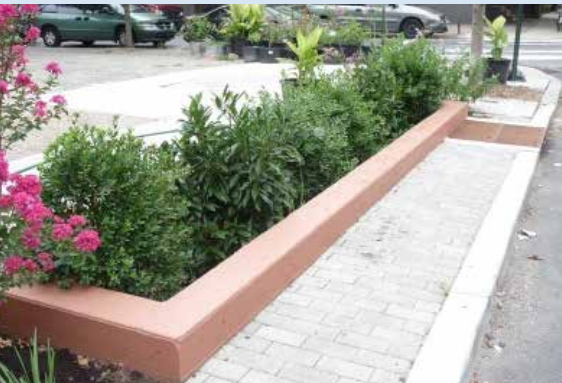
Image: Stormwater planter at Columbus Square in Philadelphia, used in part of making Reed St. a green street, via Philadelphia Water Department.
