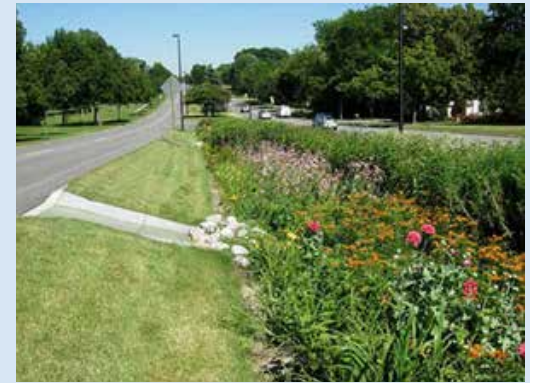
Image: Planted bioswale in Greendale, WI along a roadside, via Soil Science Society of America.
