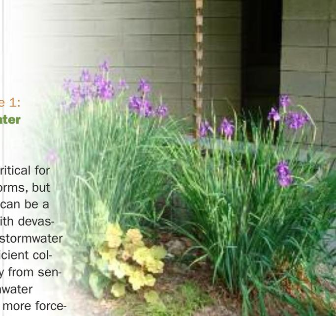
Water coming from the roof runs down this rain chain and into the planting bed.
