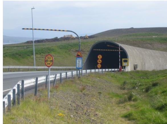
South entrance to the Hvalfjörður tunnel (Credit: Evsteinn Guðni Guðnason)
