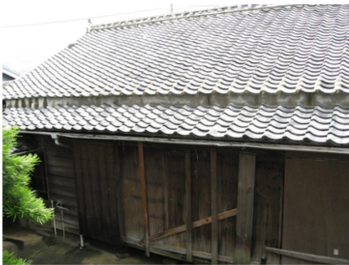
An empty house in Iwaishima (photo by the author).
