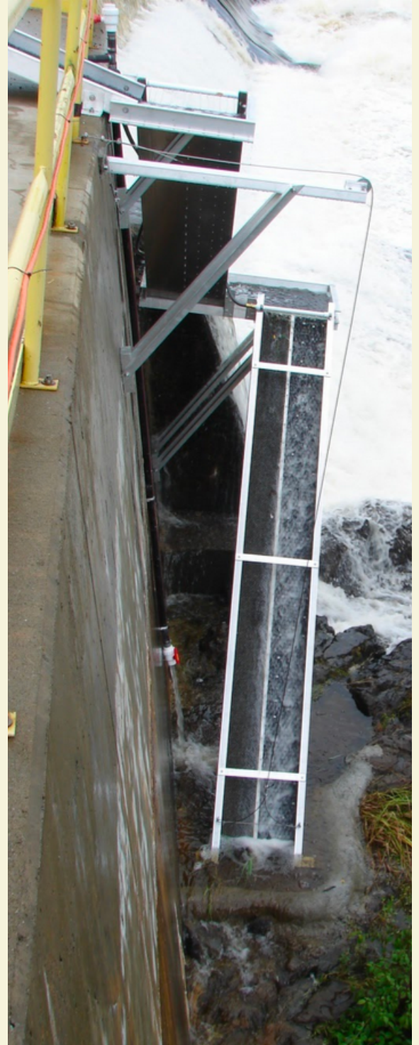
Figure 3: Typical Eel Ramp Pass (Anonymous conservationist, personal communication, February 4, 2021. Reprinted with permission.)
