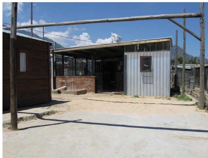
Figure 3: Outside view of the front of the WaSH facility
